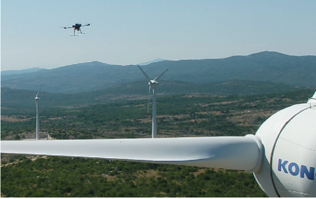
Figure 1: A multi-rotor UAV conducting an inspection of a wind turbine, capturing videos and pictures of the nacelle, rotor shaft and blades, as well as their surrounding environment, to perform a preliminary remote evaluation [3].
